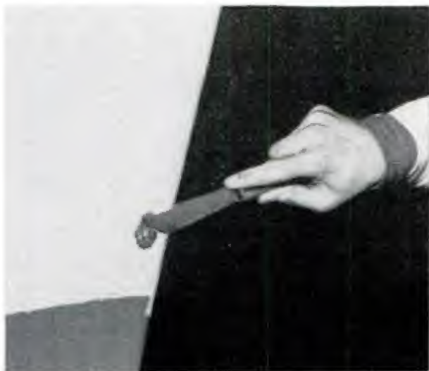
REPAIR PUTTY must have a firm seat on which to hold, so scrape away all loose distressed material
